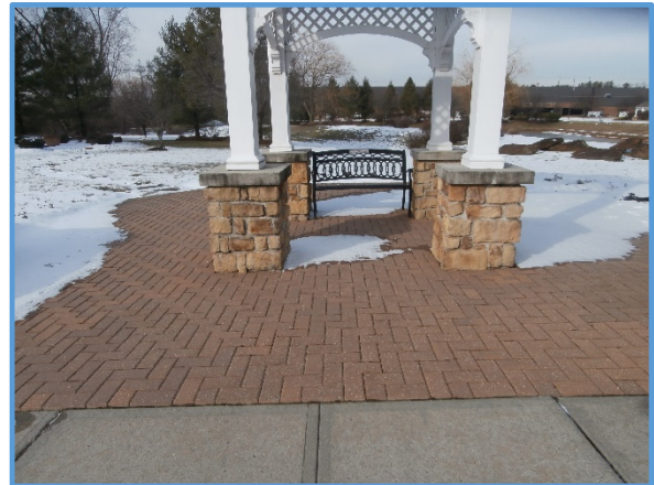
Pre-cast Concrete Paver Pad
